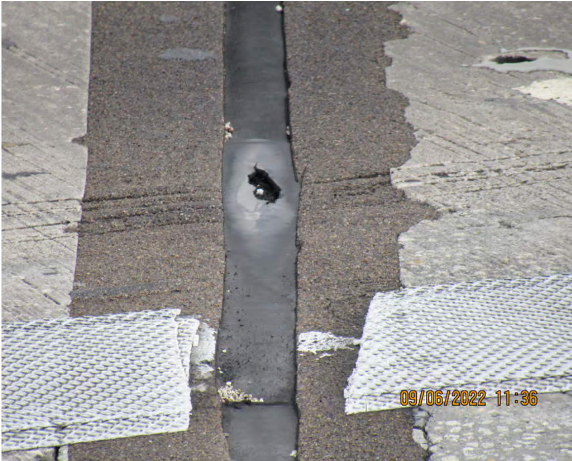
DAMAGED JOINT SEALANT (BRIDGE # 870291)
