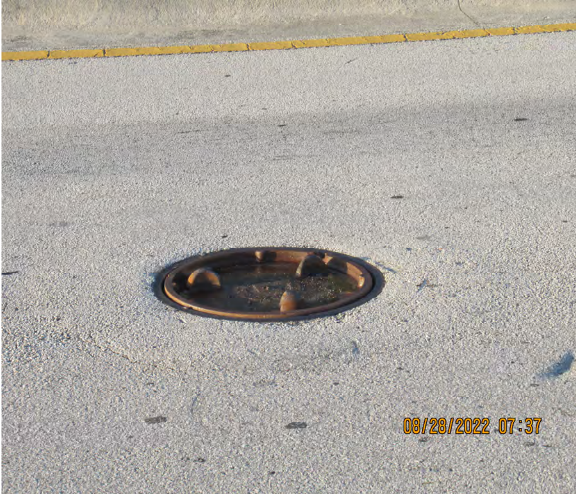
FLIPPED MANHOLE COVER
