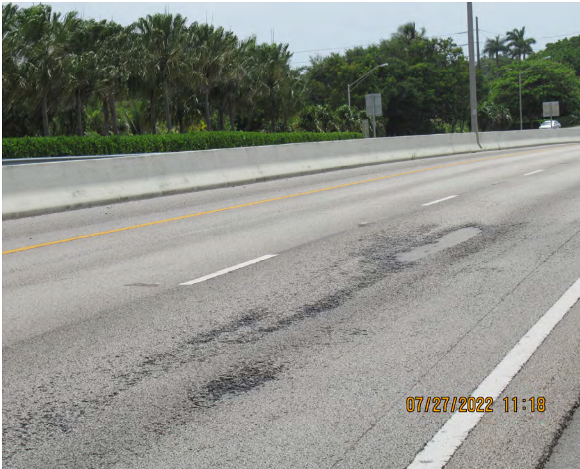
DETERIORATED PAVEMENT
