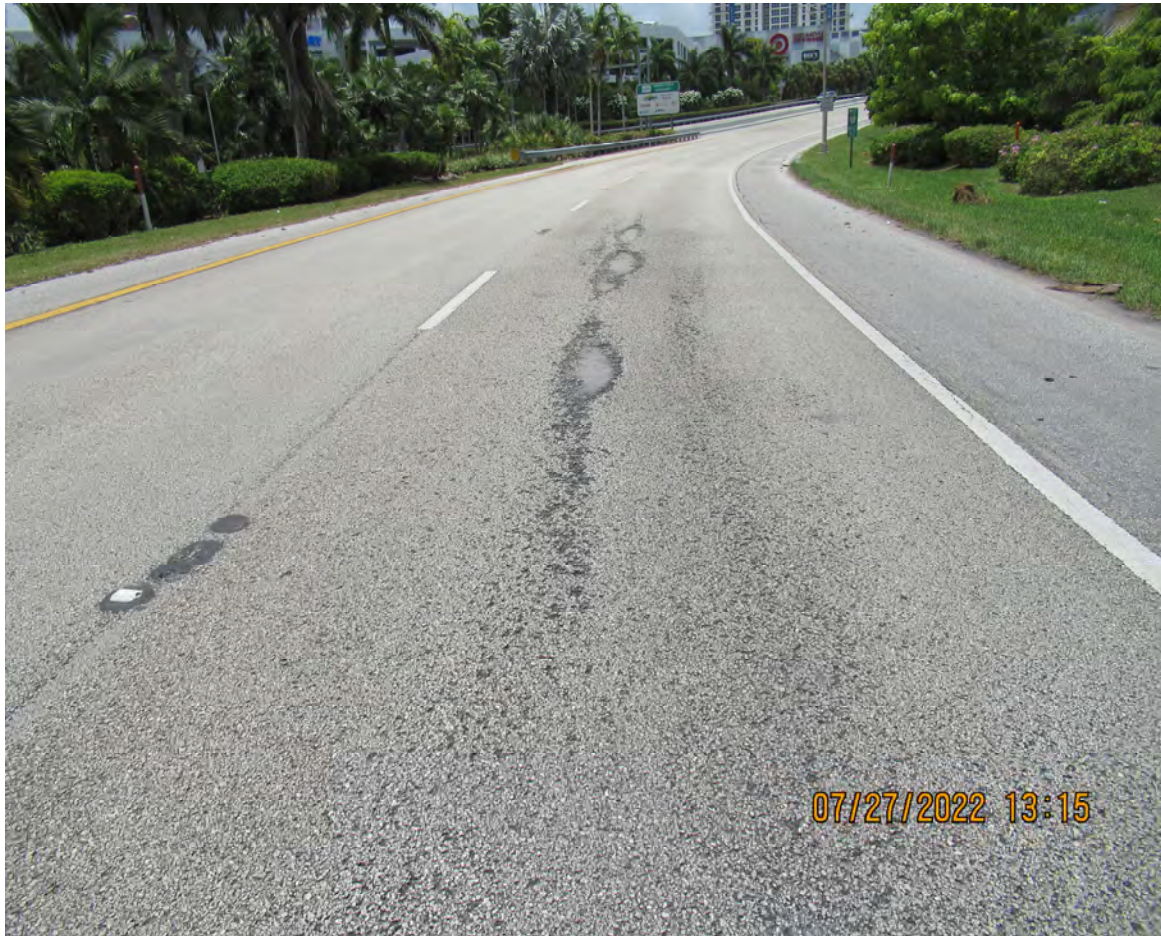
DETERIORATED ASPHALT PAVEMENT
