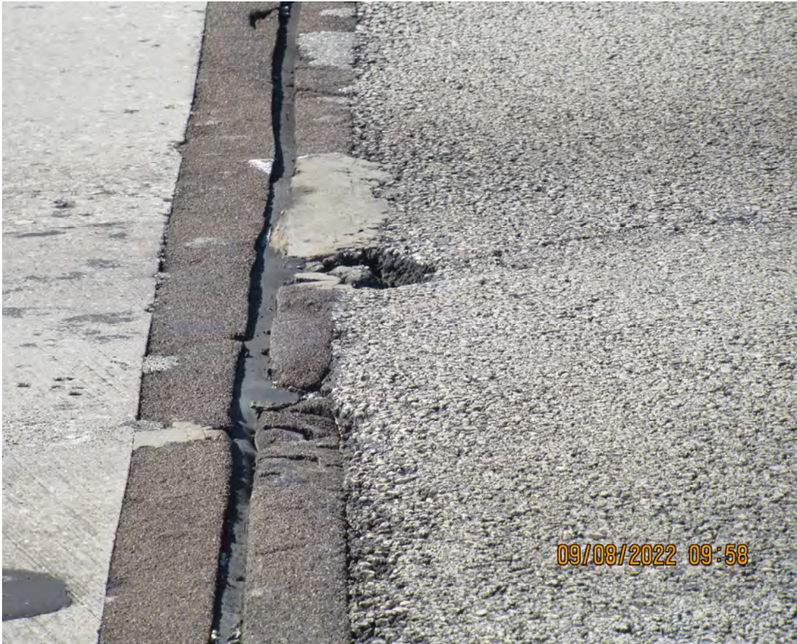
DAMAGED POLYMER NOSING JOINT HEADER (BRIDGE # 870138)
