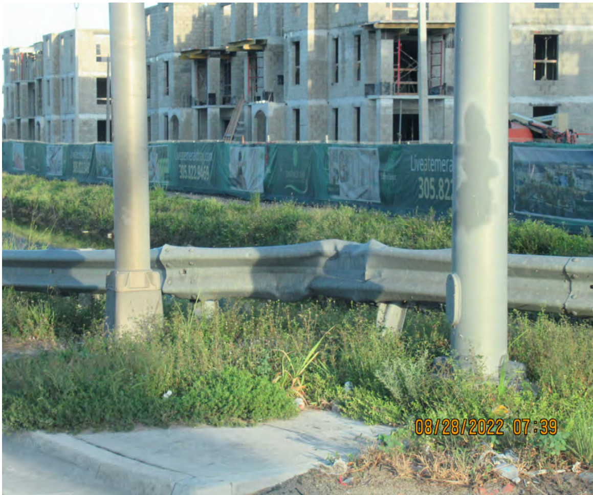
DAMAGED GUARDRAIL
