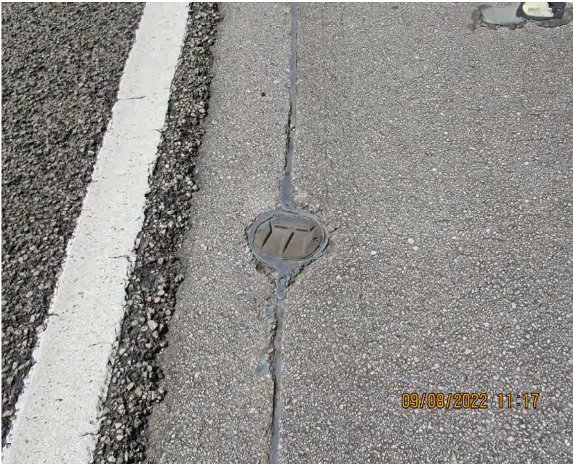
MALFUNCTIONING ILLUMINATED REFLECTIVE PAVEMENT MARKERS
