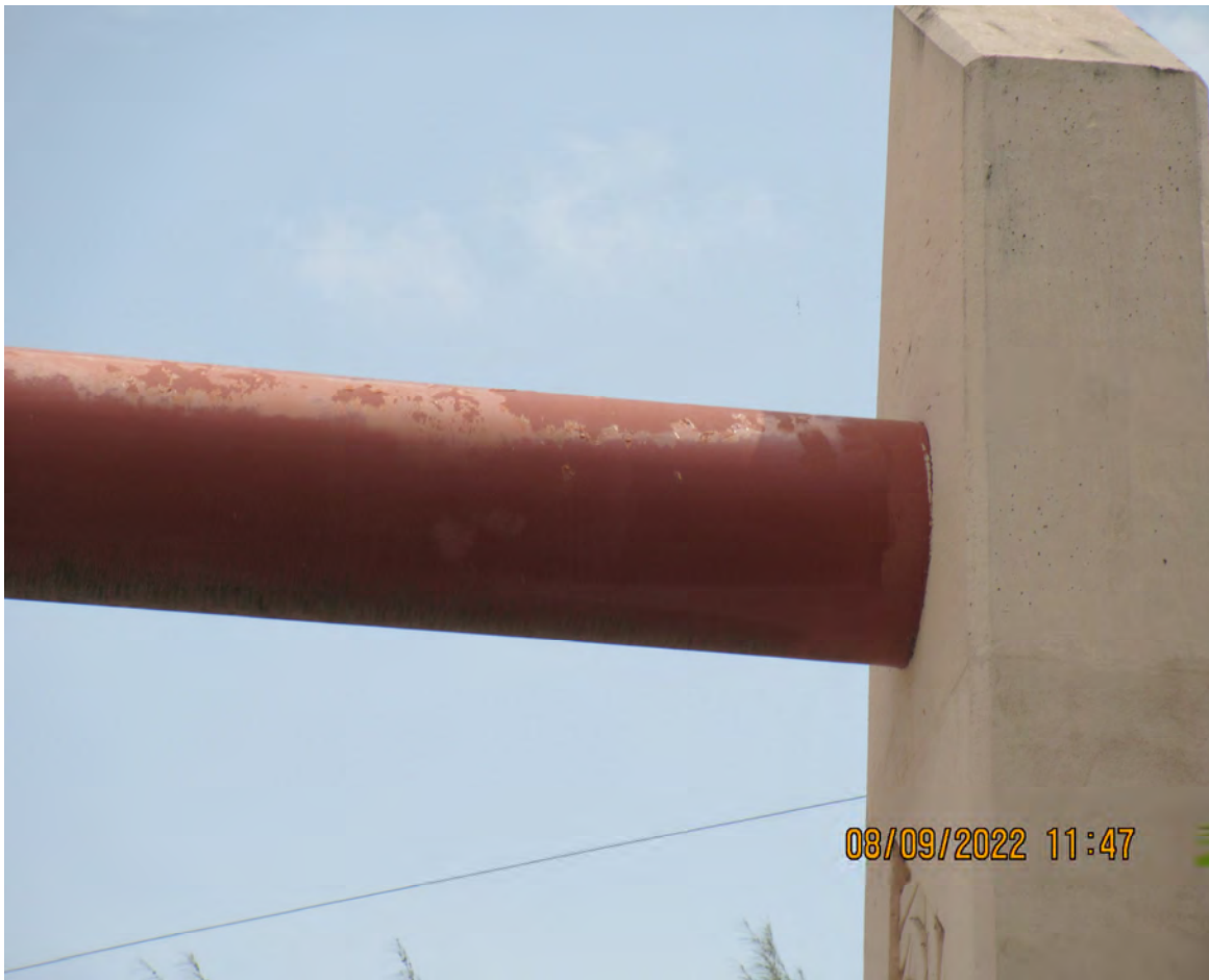
DETERIORATED PAINT ON MONOTUBE (STRUCTURE # 87A134)
