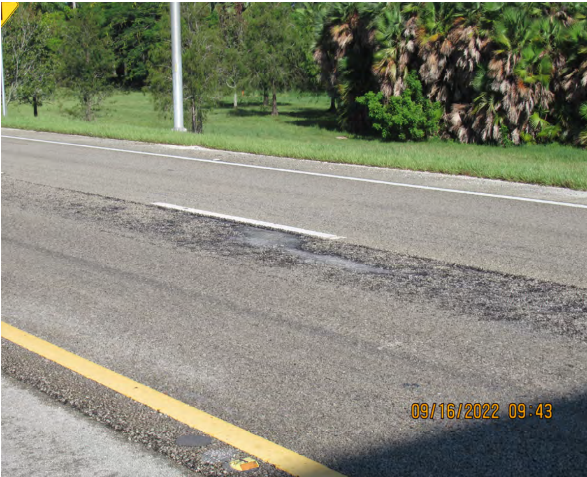
DETERIORATED PAVEMENT
