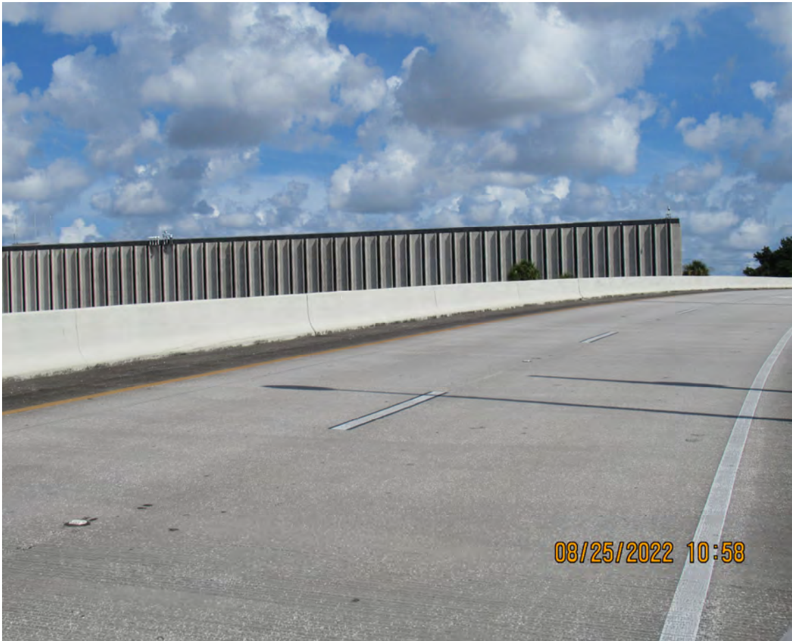
DETERIORATED EDGELINE STRIPING (BRIDGE No. 870726)
