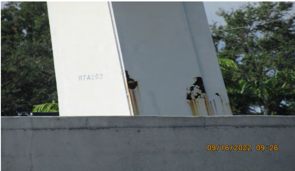
CORROSION ON PILONS (STRUCTURE # 87A253)
