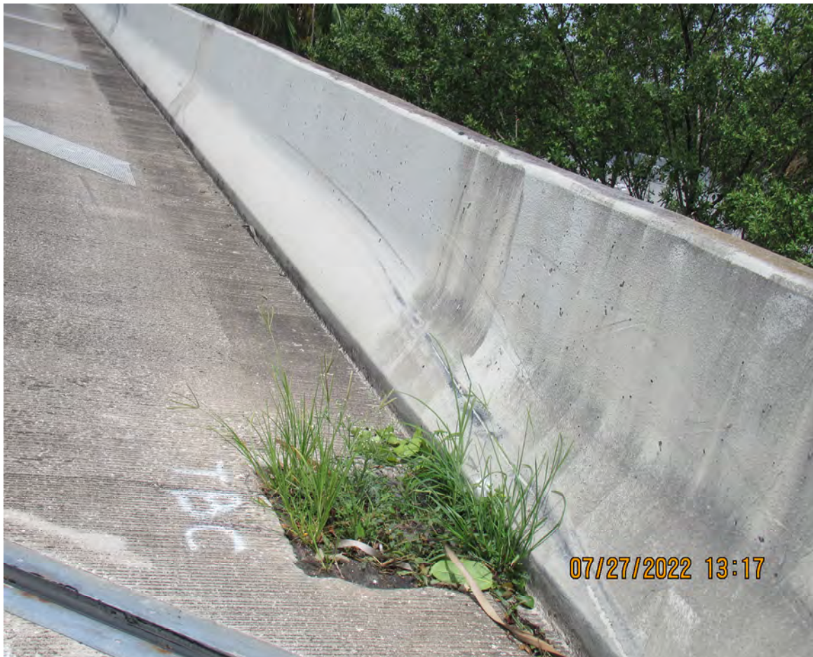
SILTED DECK DRAINS (TYPICAL AT VARIOUS LOCATIONS)
