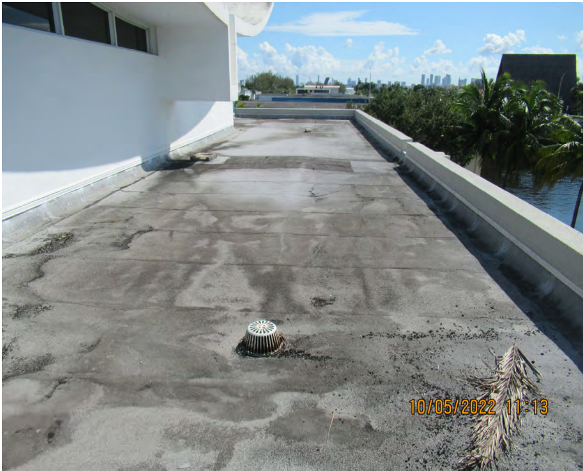
BLISTERING ON THE ROOFING MEMBRANE
