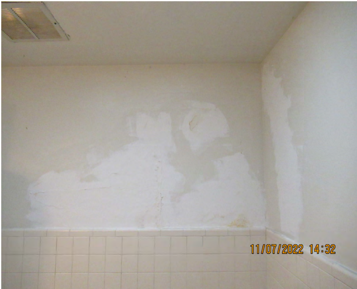
UNFINISHED DRYWALL REPAIRS IN BATHROOM WALLS
