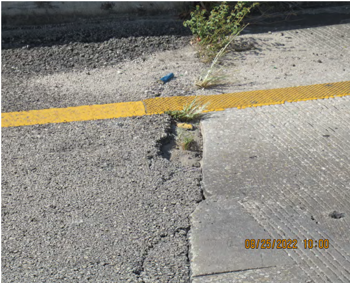
DETERIORATED ASPHALT PAVEMENT AT BENT #2 (BRIDGE # 870122)
