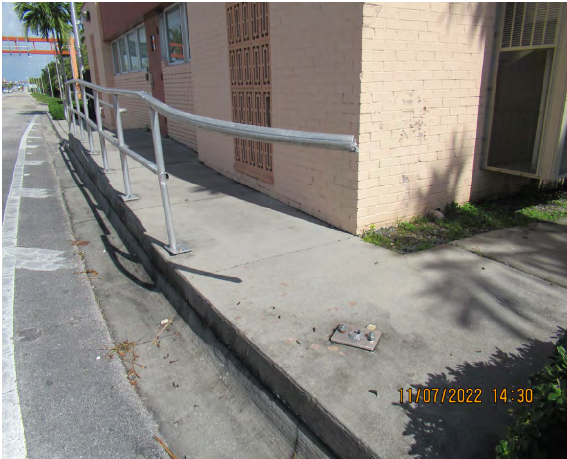
DAMAGED PEDESTRIAN RAILING
