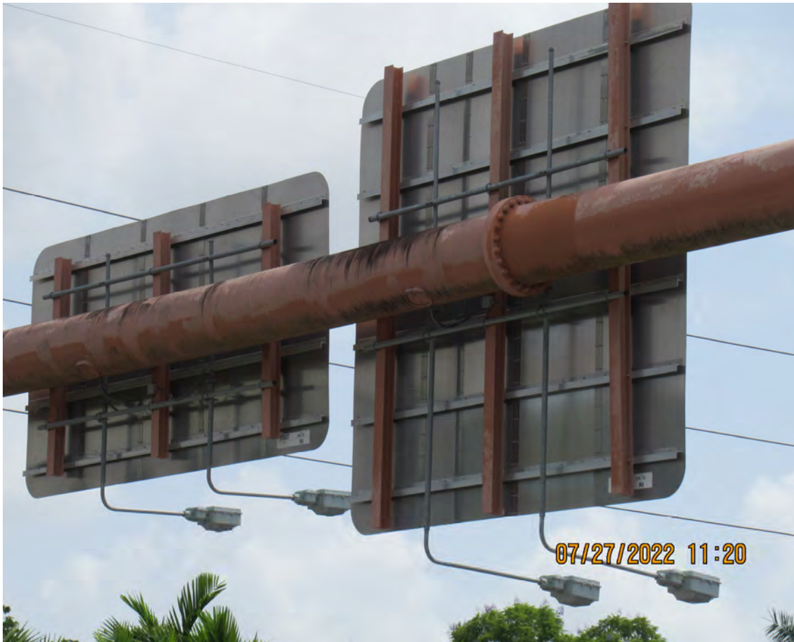
DETERIORATED PAINT ON MONOTUBE
