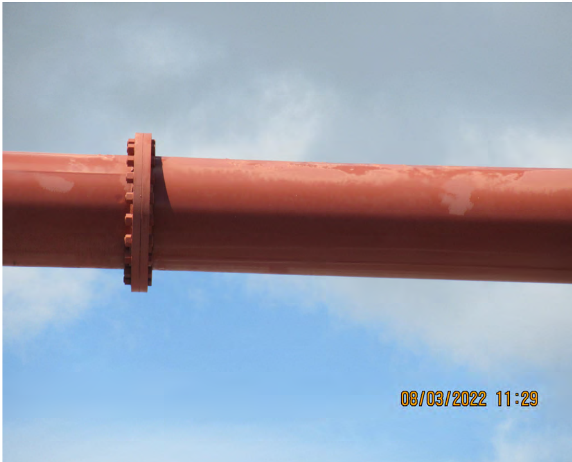
DETERIORATED PAINT ON MONOTUBE (STRUCTURE # 87A130)
