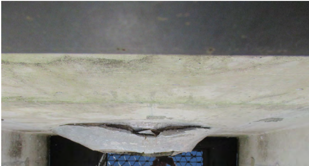
DETERIORATED PIPE SEAL
