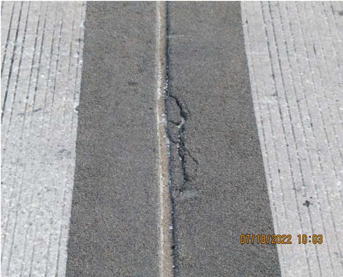
DETERIORATED EXPANSION JOINT HEADER (BRIDGE # 870720)
