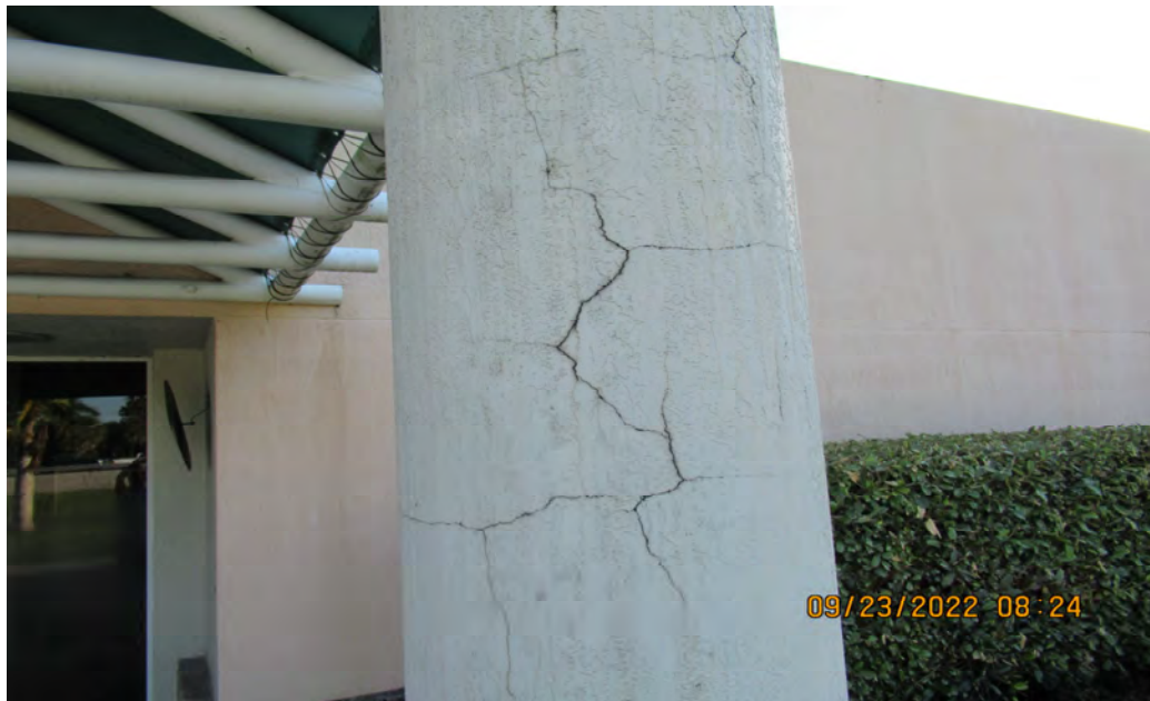
CRACKS ON STUCCO
