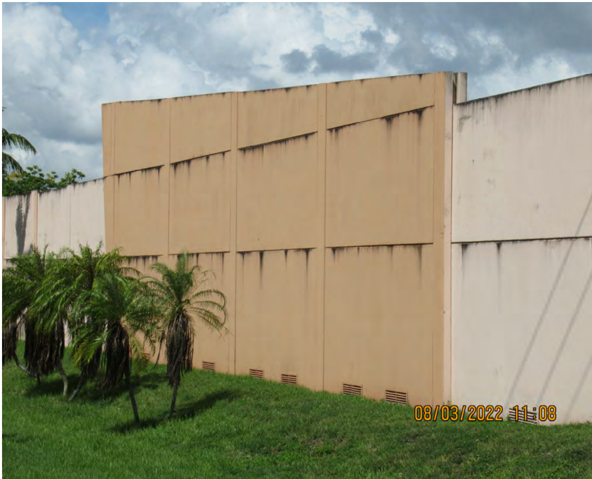
DETERIORATED CLASS V COATING ON SOUND WALL (TYPICAL AT VARIOUS LOCATIONS)
