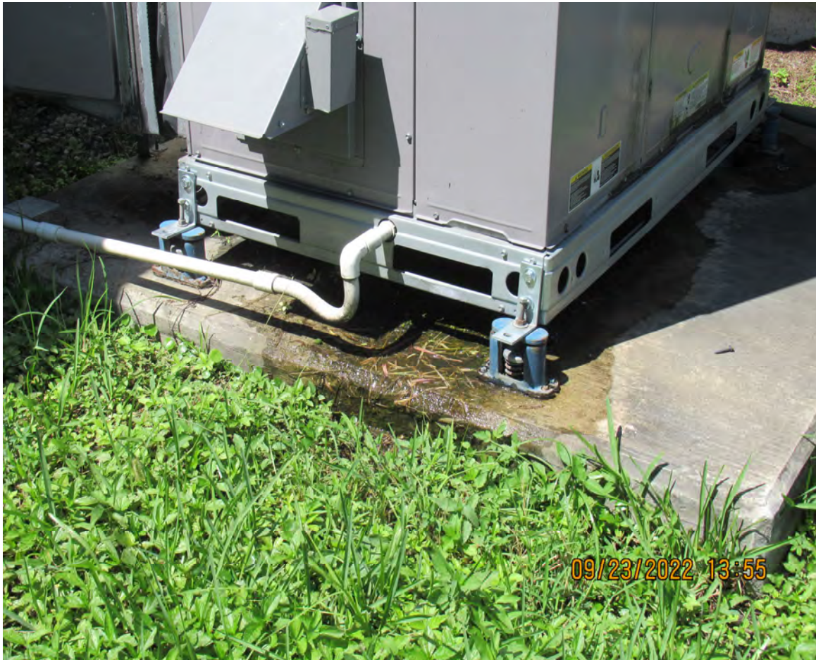
CLOGGED CONDENSATE DRAIN (TYPICAL OF BOTH HVAC UNITS)
