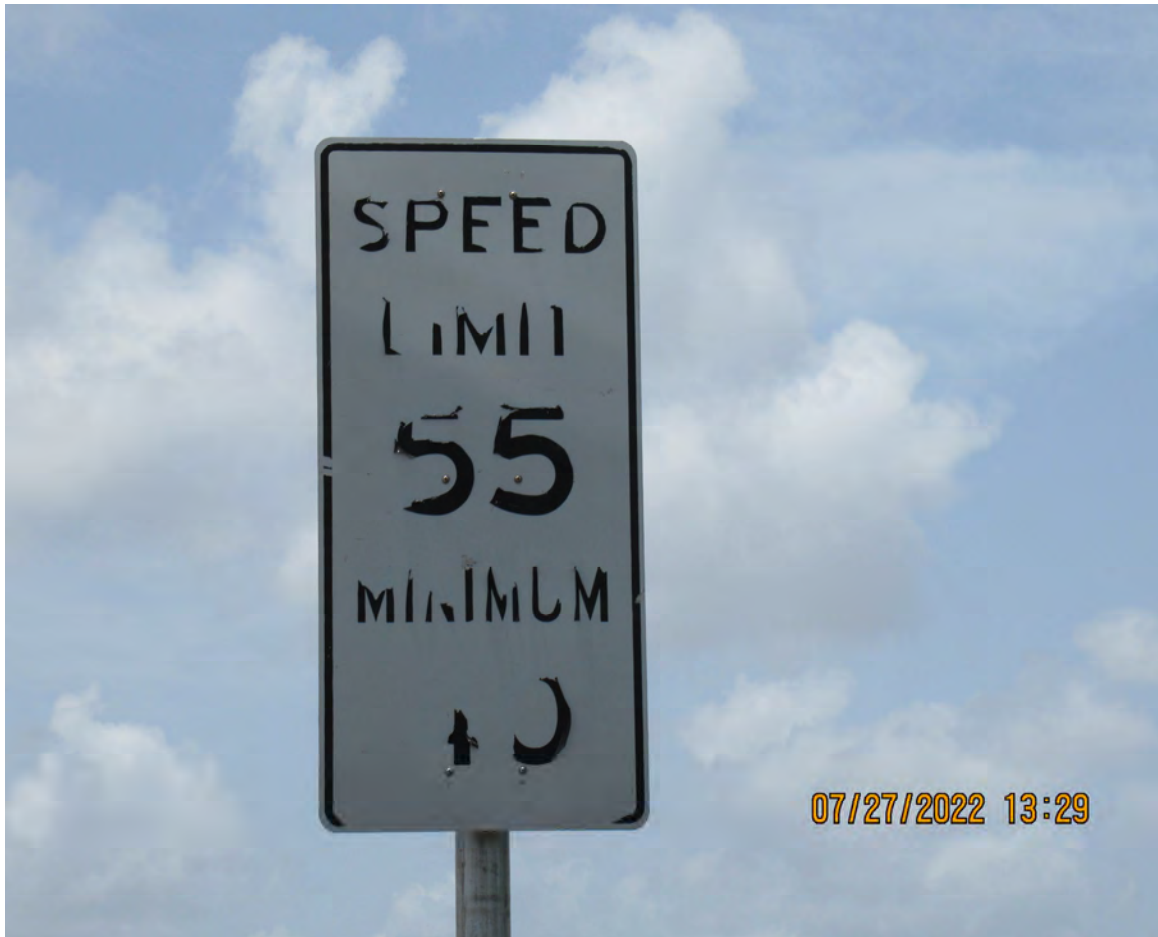
DETERIORATED REFLECTIVE SHEETING
