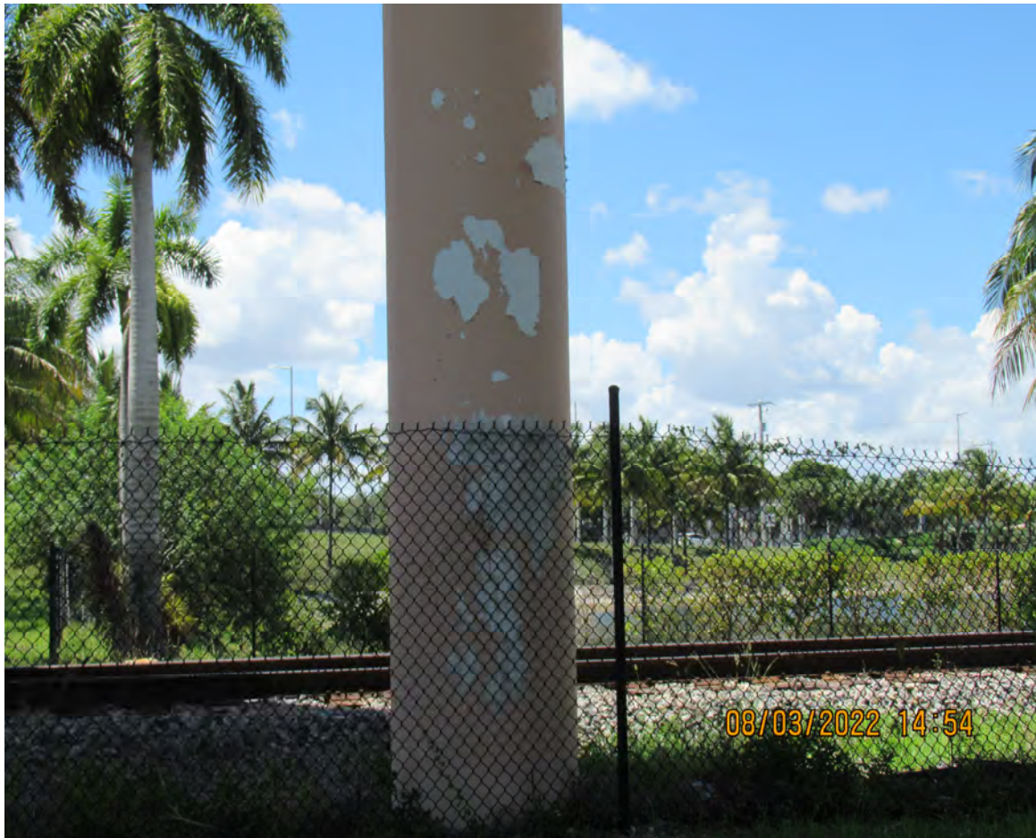
DETERIORATED CLASS V COATING ON BRIDGE COLUMNS
