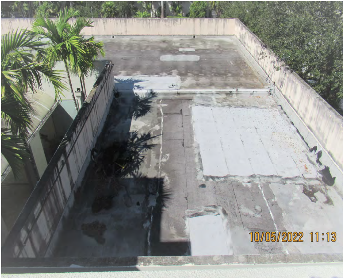
MISSING INSULATION ON REFRIGERANT LINE
