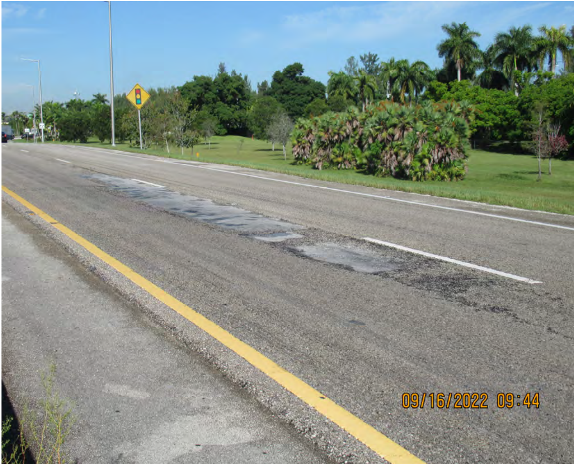
DETERIORATED PAVEMENT
