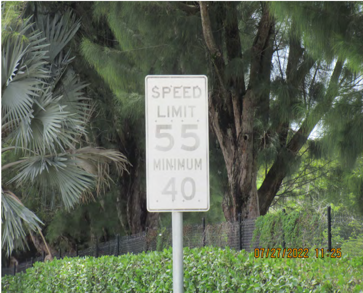
DETERIORATED REFLECTIVE SHEETING
