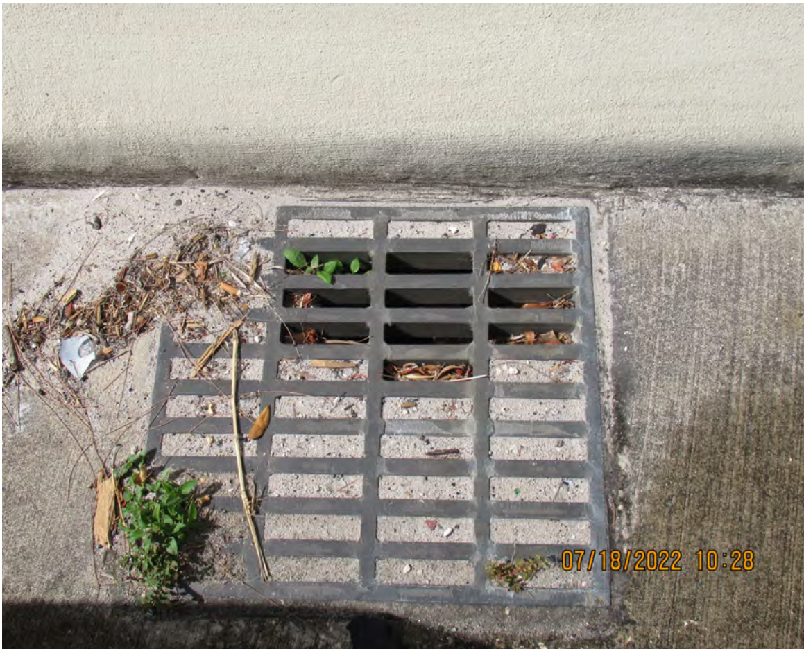
SILTED BRIDGE DECK DRAIN
