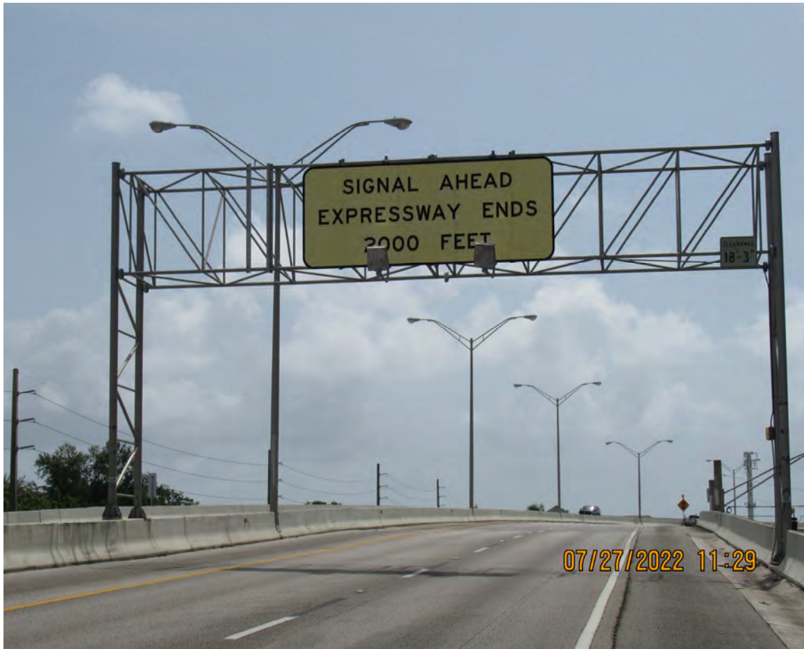
DETERIORATED REFLECTIVE SHEETING
