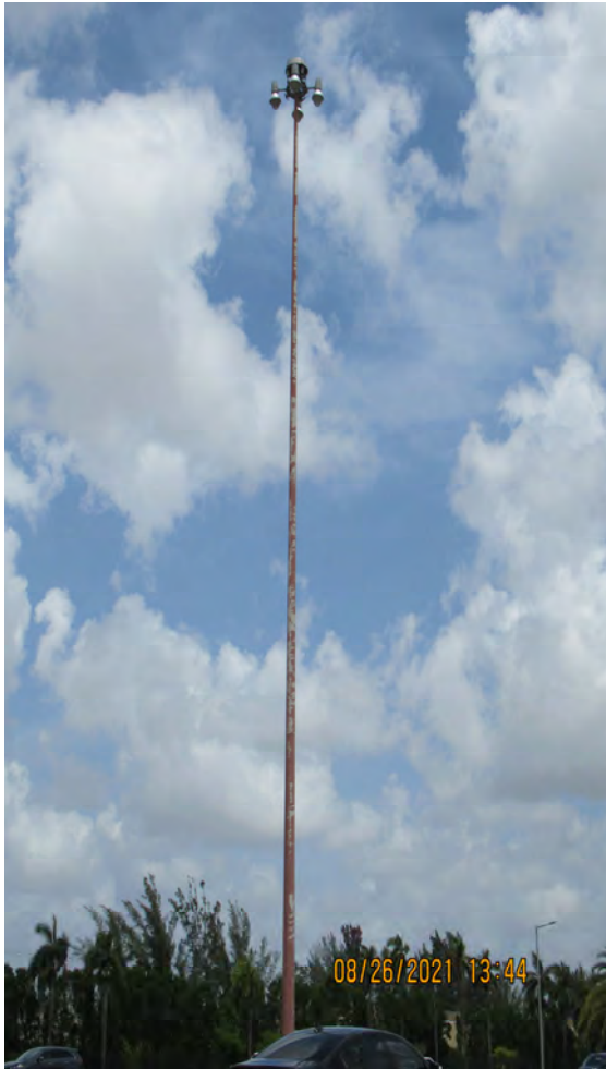
DETERIORATED PAINT ON HIGH MAST LIGHT POLE
