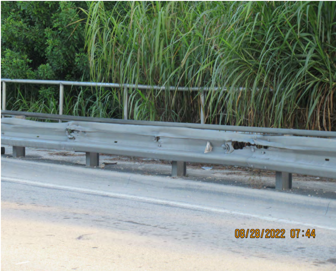
DAMAGED GUARDRAIL
