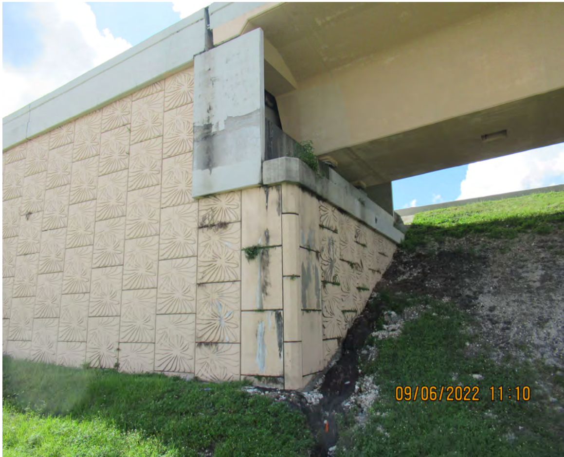
DETERIORATED CLASS V COATING AT BENT 12 (BRIDGE # 871050)
