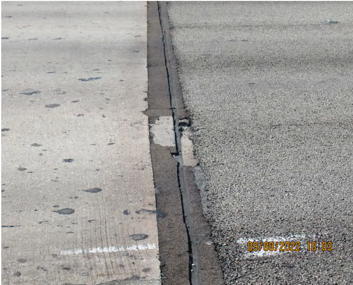
DAMAGED POLYMER NOSING JOINT HEADER (BRIDGE # 870137)
