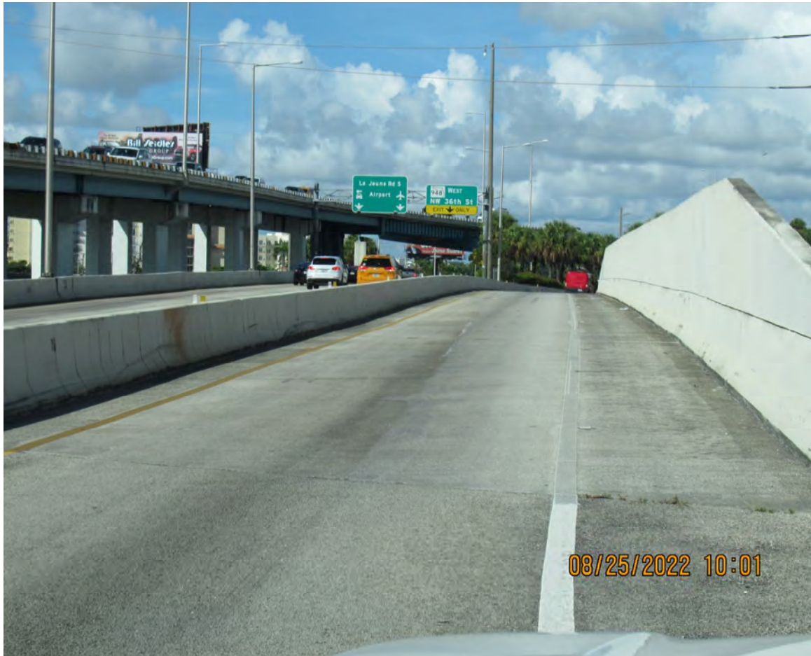
DETERIORATED STRIPING ON BRIDGE (BRIDGE # 870026)
