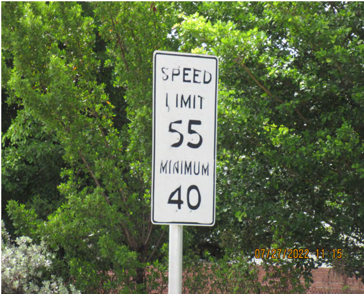
DETERIORATED REFLECTIVE SHEETING
