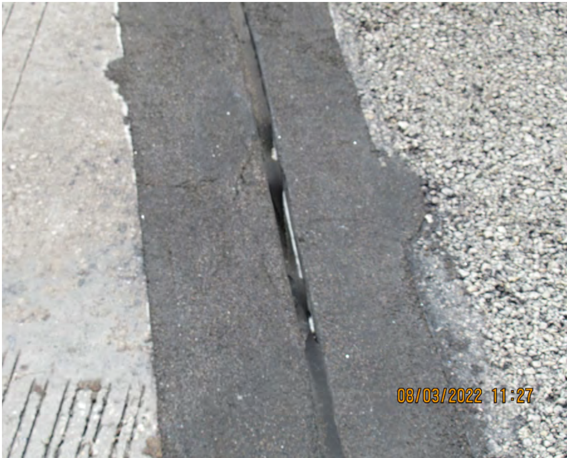
DETERIORATED JOINT SEALANT BENT 1 (BRIDGE # 870495)
