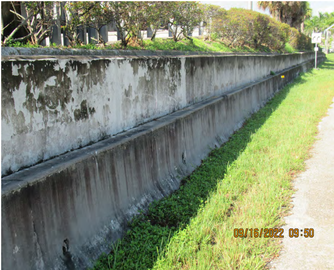
DETERIORATED CLASS V COATING ON RETAINING WALL
