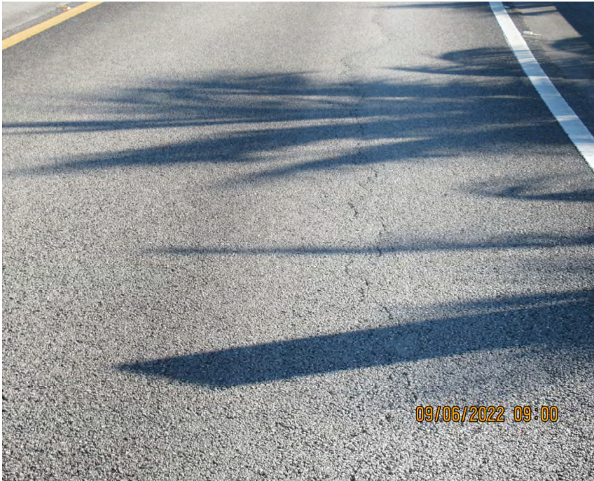
LONGITUDINAL CRACK ON PAVEMENT
