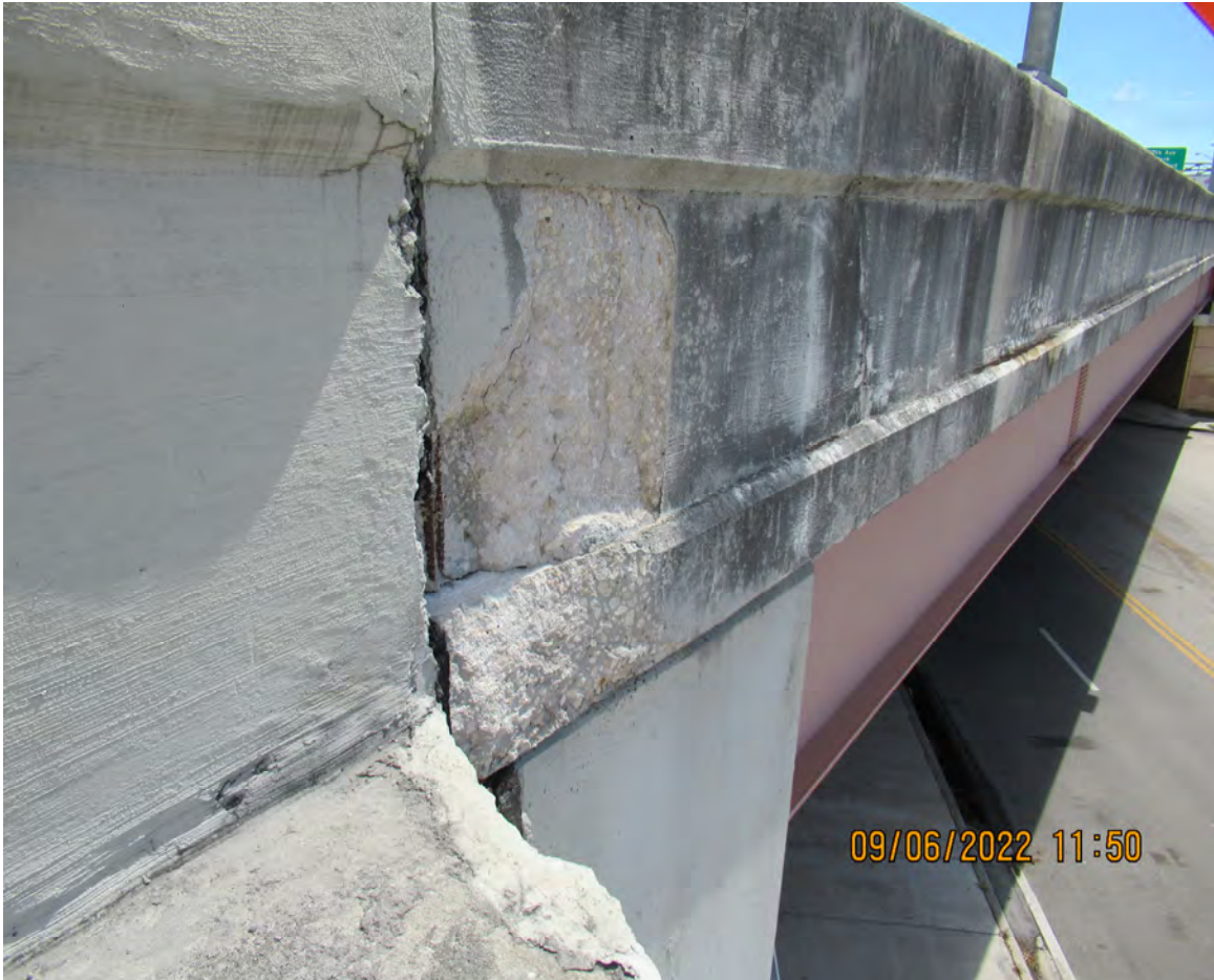
SPALLS ON ABUTMENT 1 TRAFFIC RAILING AND SLAB (BRIDGE # 870966)
