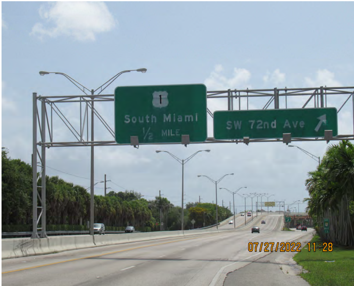
DETERIORATED REFLECTIVE SHEETING
