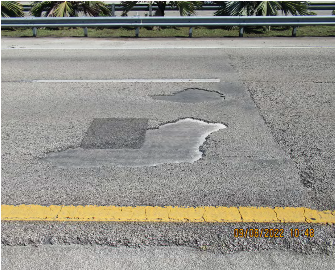
DAMAGED FRICTION COURSE PAVEMENT
