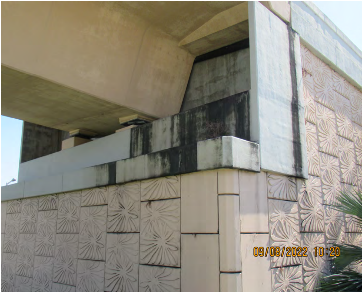
WATER STAINS FROM CLOGGED JOINT DRAINAGE (BRIDGE # 871046)
