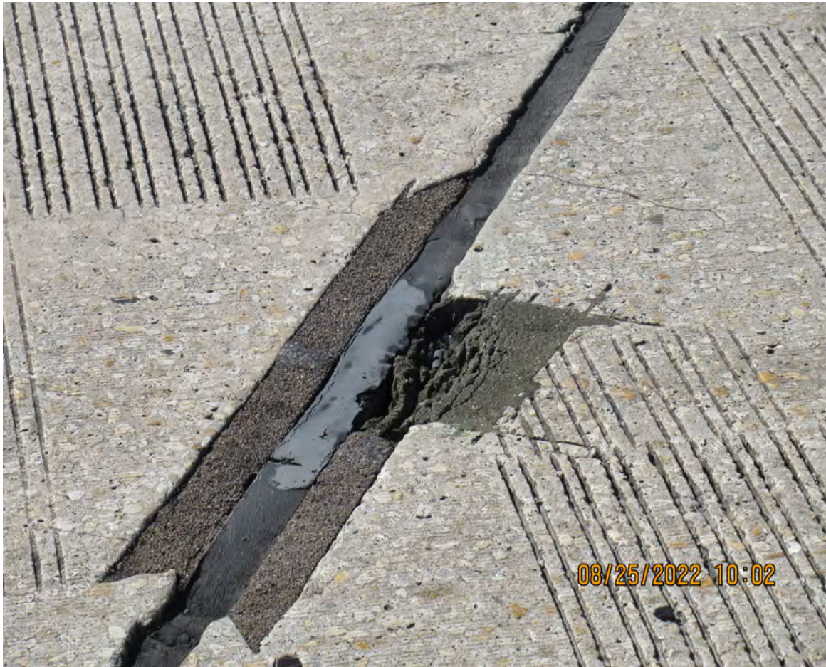
DETERIORATED JOINT REPAIR (BRIDGE # 870026)
