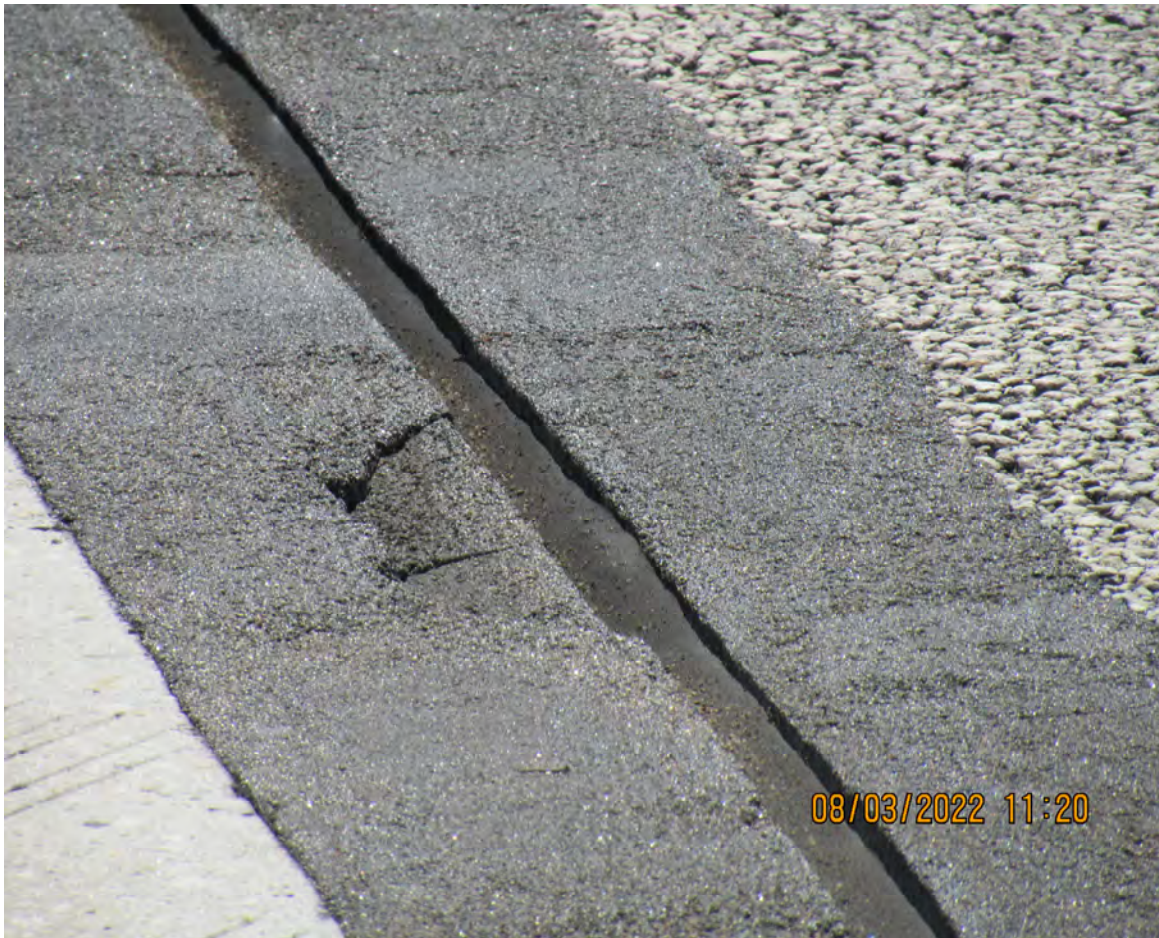
DETERIORATED POLYMER NOSING JOINT HEADER BENT 1 (BRIDGE # 870522)
