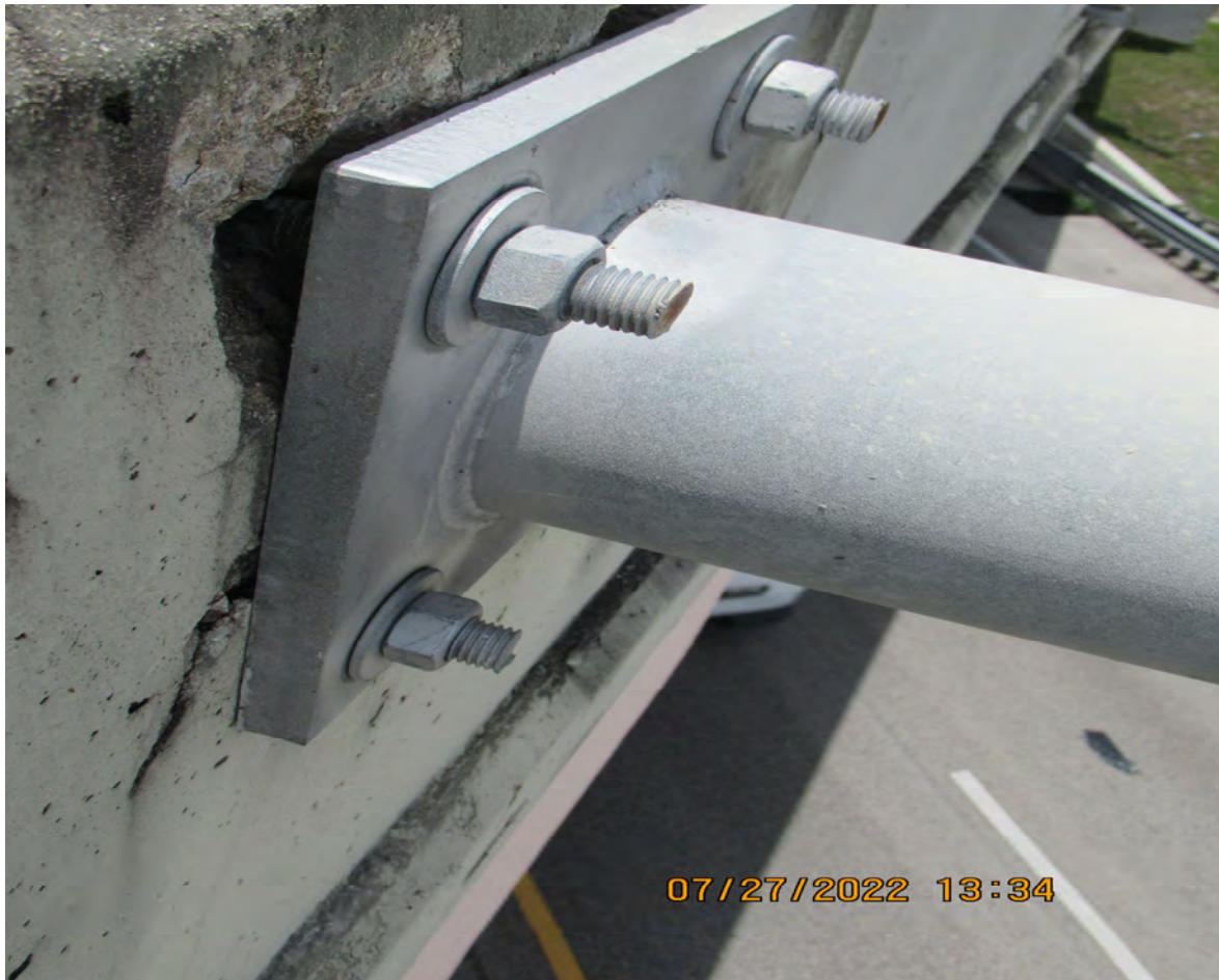
SPALL ON BACKSIDE OF TRAFFIC RAILING
