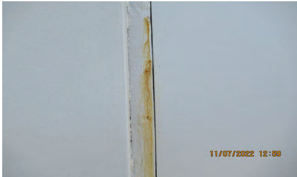
CORROSION ON METAL DOOR FRAME
