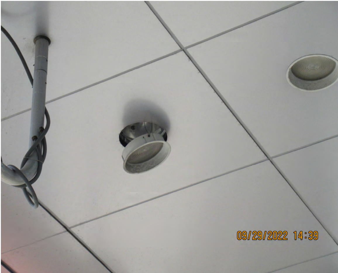
HANGING RECESSED LUMINAIRE
