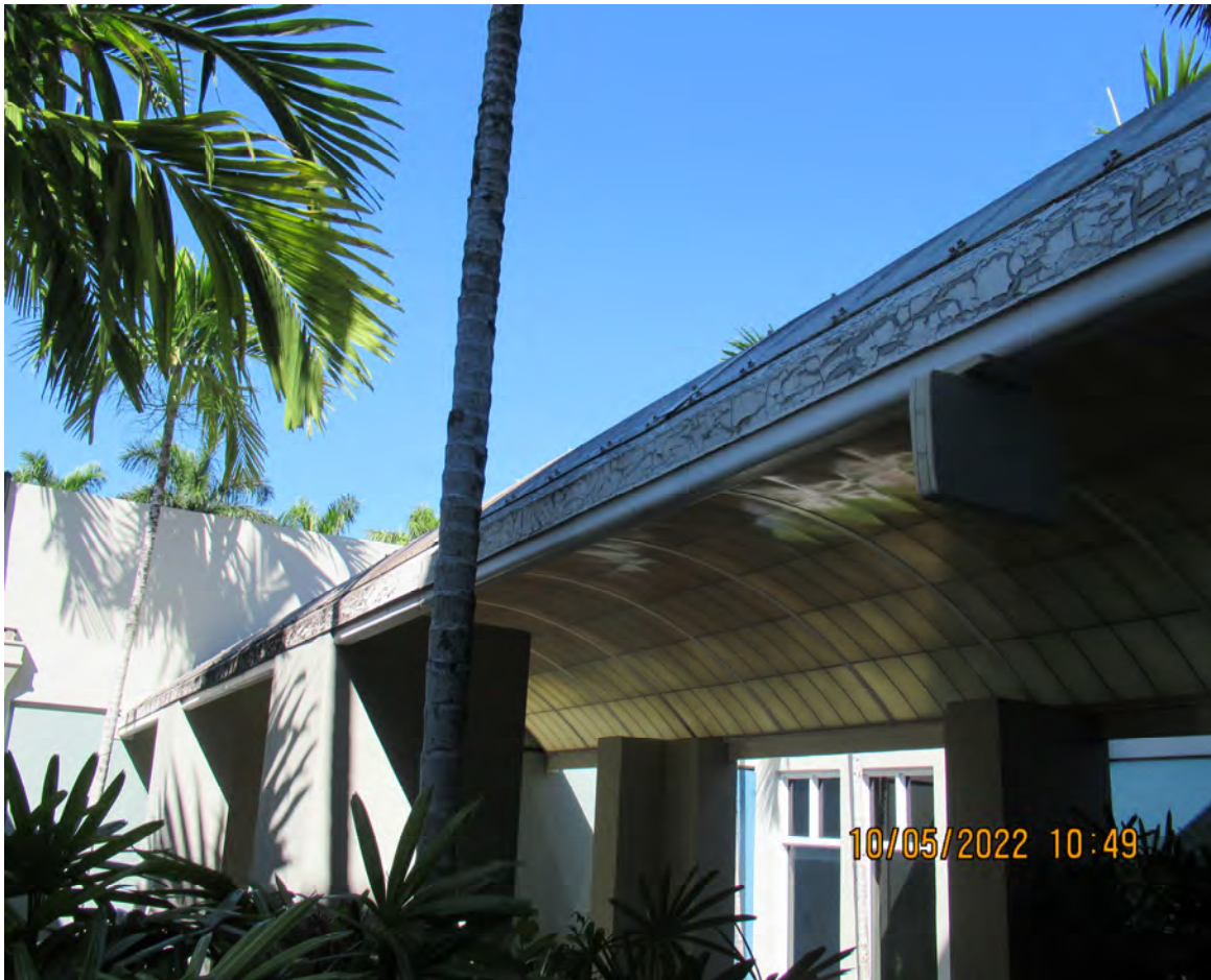
DETERIORATED PAINT ON CANOPY FRAME
