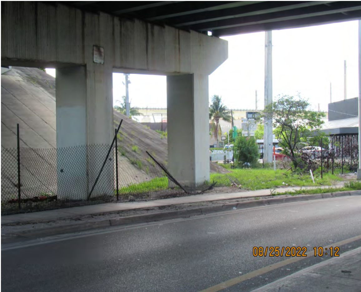
DAMAGED FENCE UNDERNEATH BRIDGE # 870238
