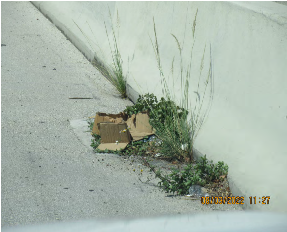
SILTED DRAINAGE STRUCTURE
