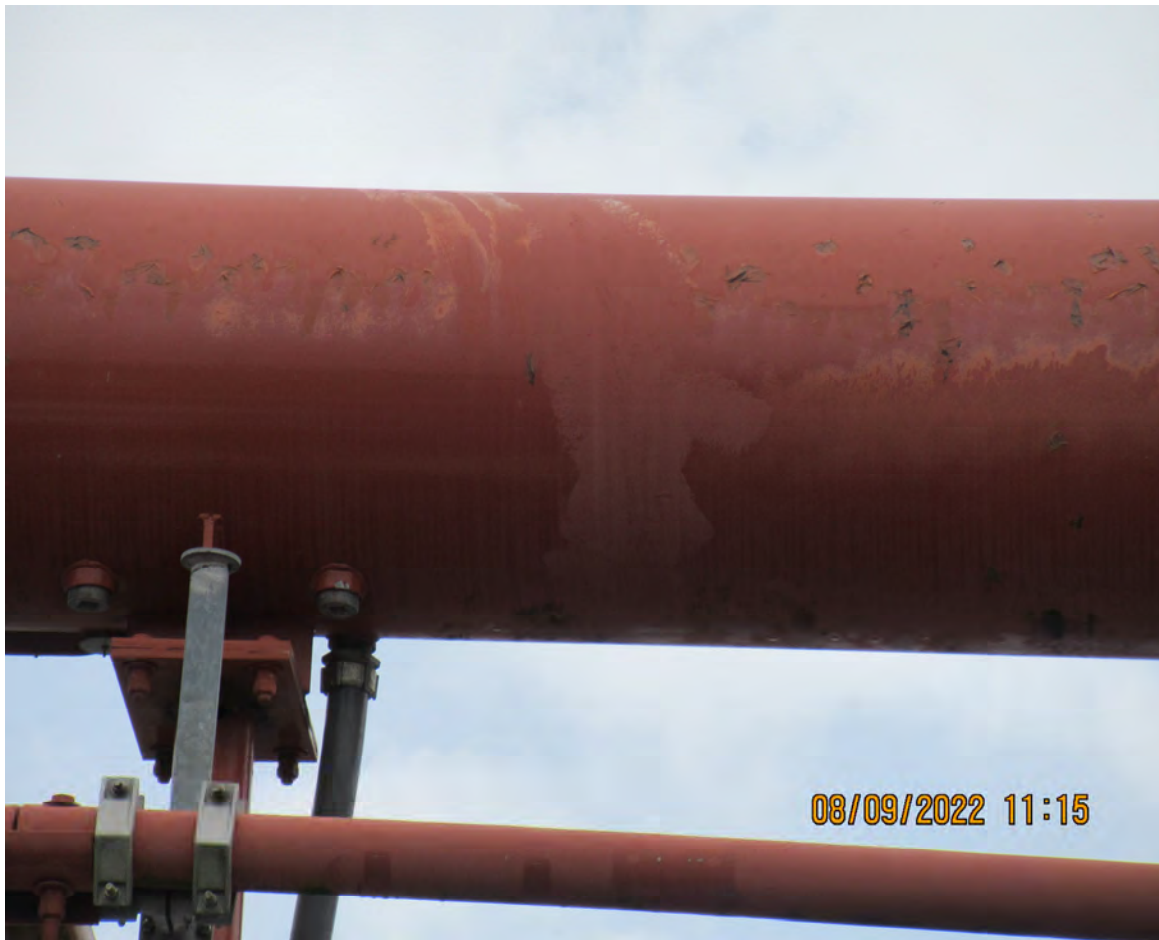
DETERIORATED PAINT ON ORT GANTRY MONOTUBE (STRUCTURE # 87S937)
