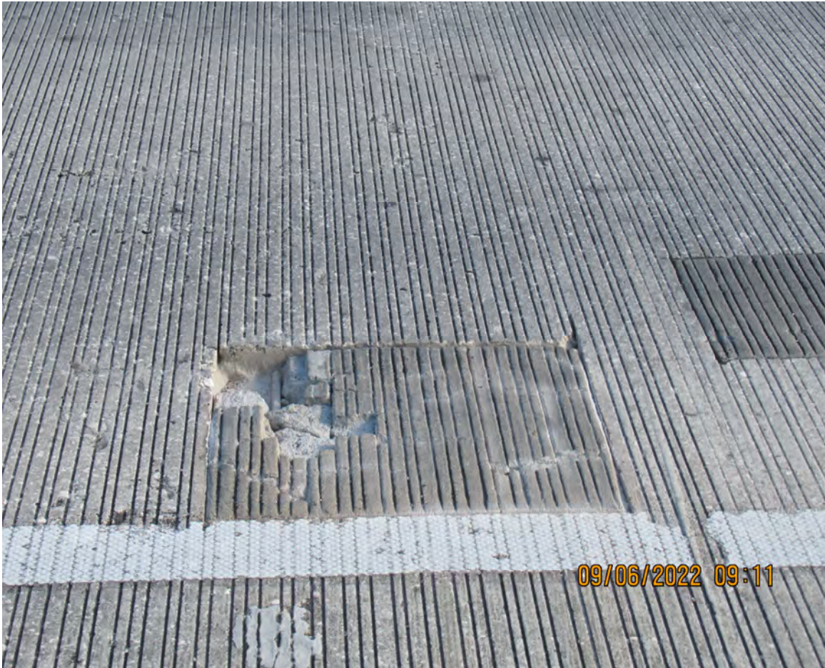
SPALL ON BRIDGE DECK (BRIDGE No. 871002)
