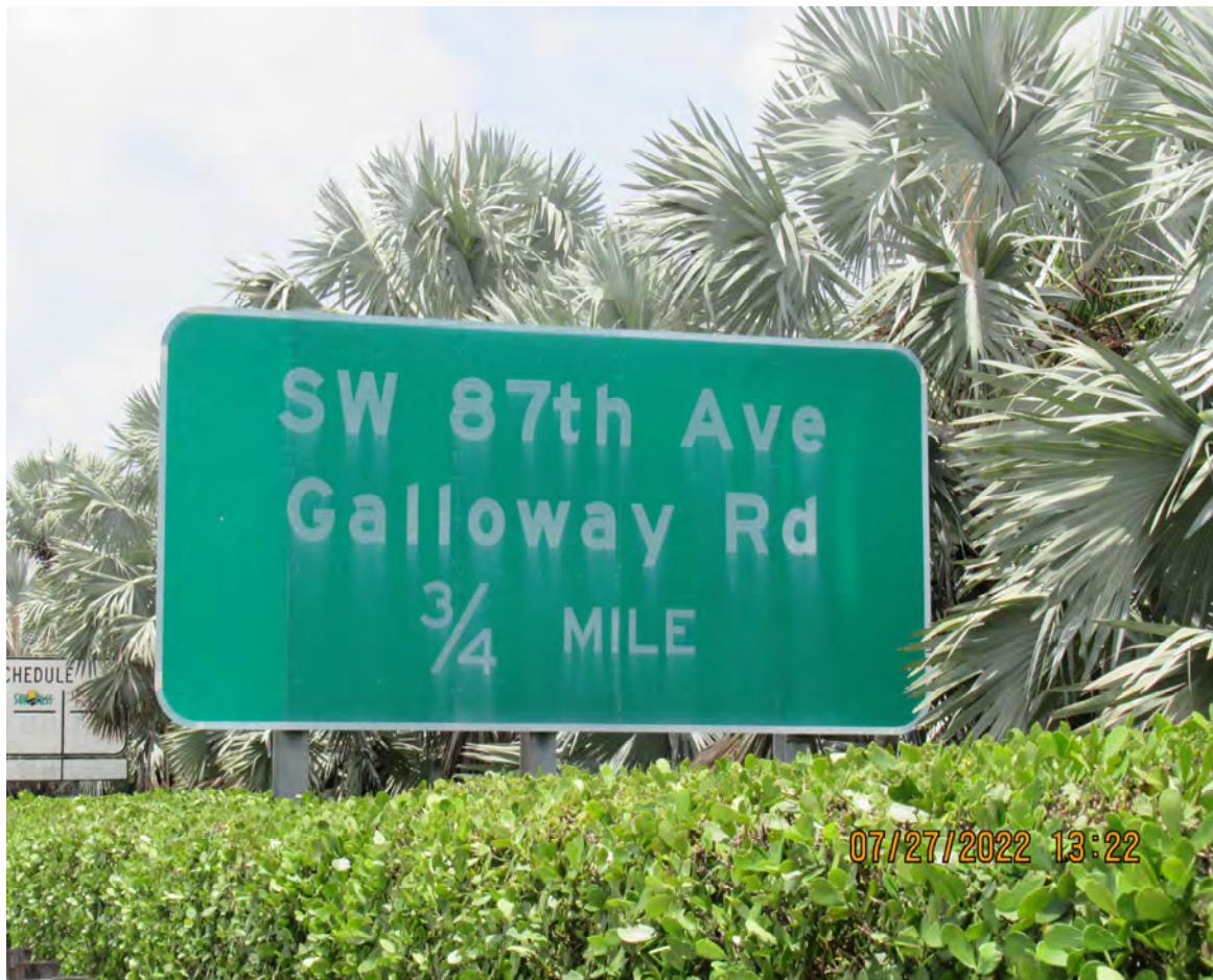
DETERIORATED REFLECTIVE SHEETING
