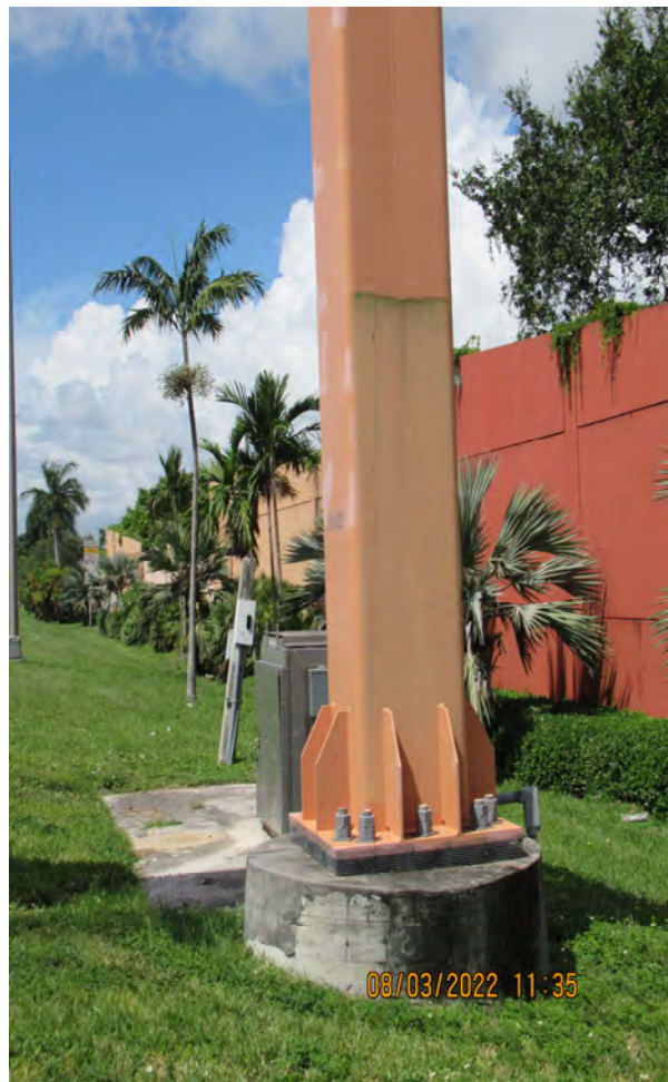
DETERIORATED PAINT ON MONOTUBE (STRUCTURE # 87A327)
