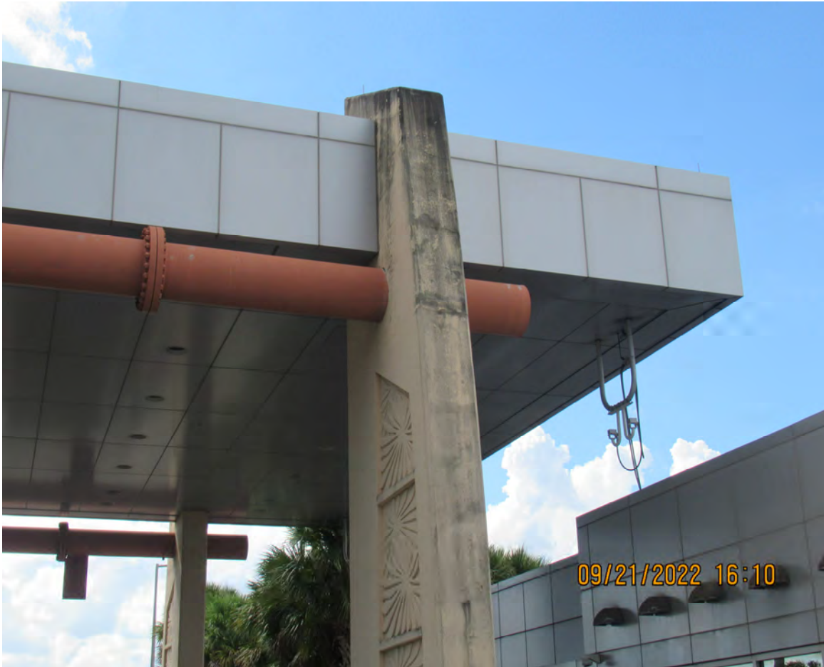
DETERIORATED CLASS 5 COATING ON CANOPY COLUMNS
