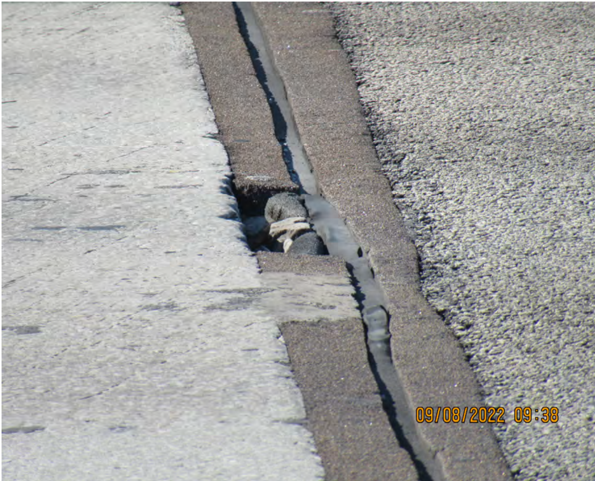
DAMAGED POLYMER NOSING JOINT HEADER (BRIDGE No. 870140)
