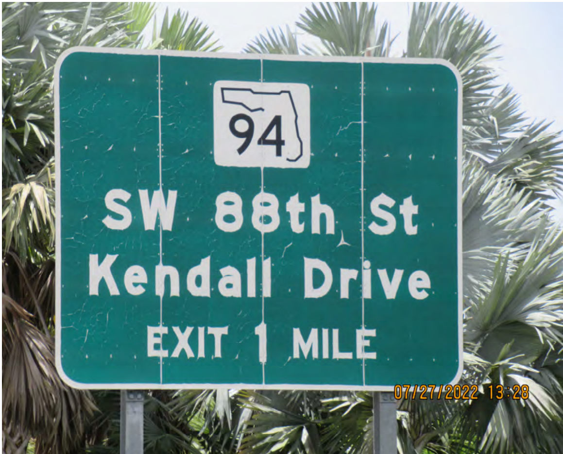
DETERIORATED REFLECTIVE SHEETING
