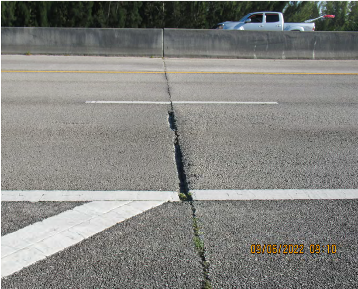
TRANSVERSE CRACK ON PAVEMENT AT APPROACH SLAB (BRIDGE No. 871002)
