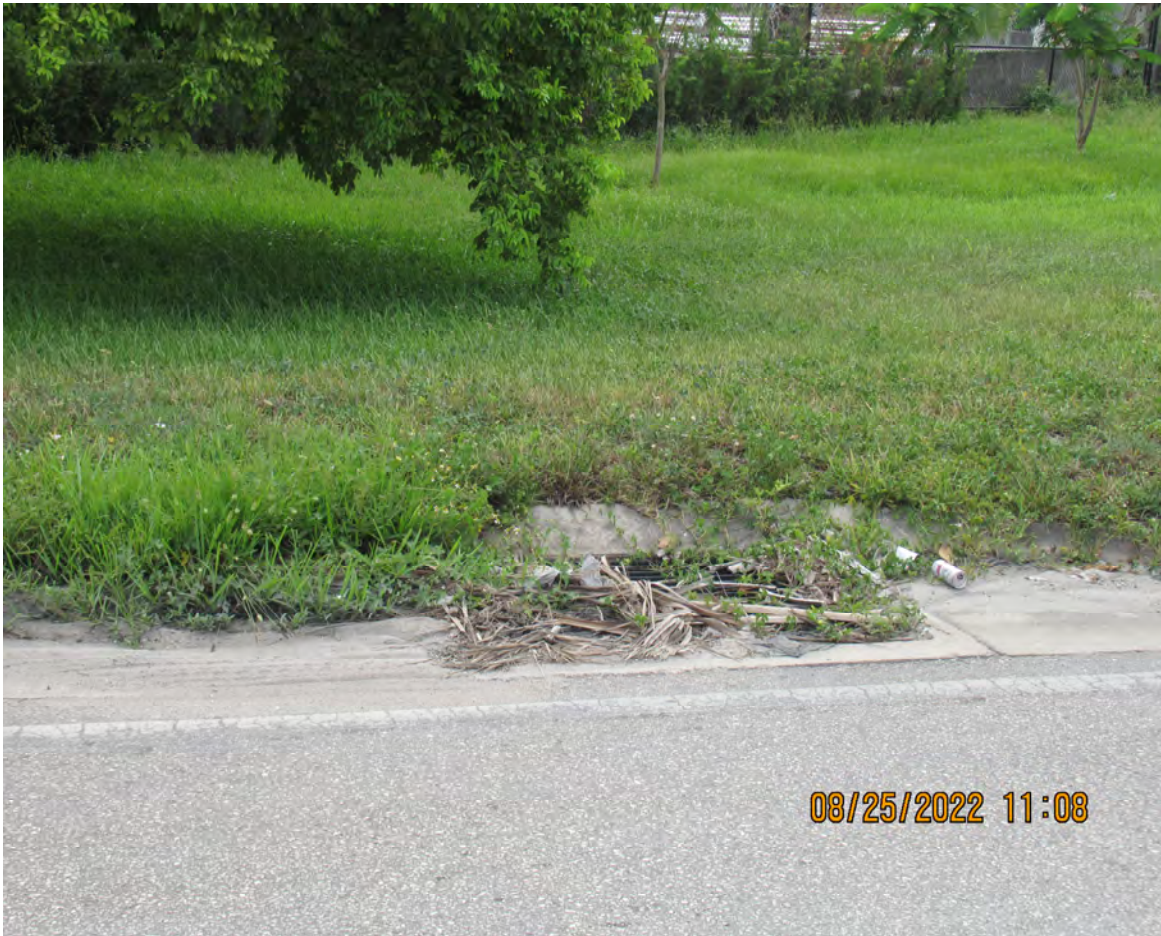
SILTED DRAINAGE STRUCTURE
