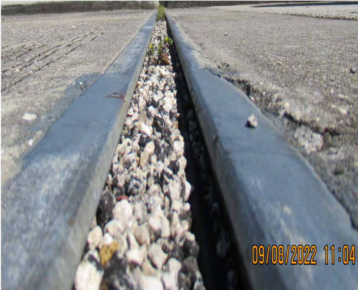
DEBRIS ON BRIDGE EXPANSION JOINT (BRIDGE No. 871008) (TYPICAL THROUGHOUT)
