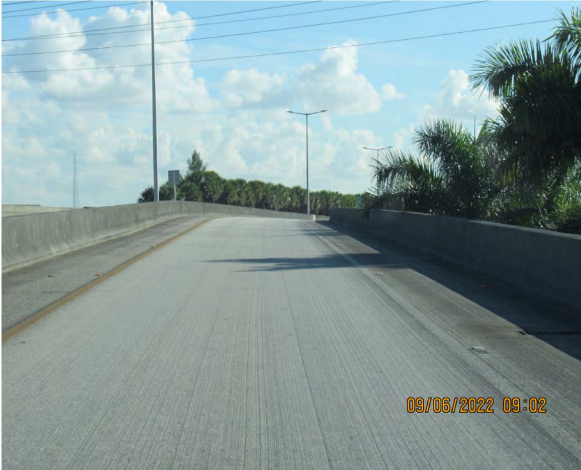
DETERIORATED STRIPING (BRIDGE No. 871008)
