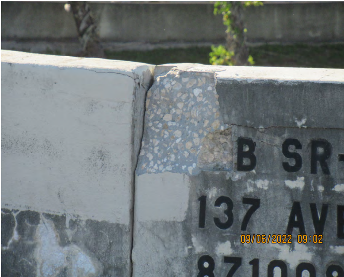
SPALL ON TRAFFIC RAILING (ABUTMENT 1, BRIDGE No. 871008)
