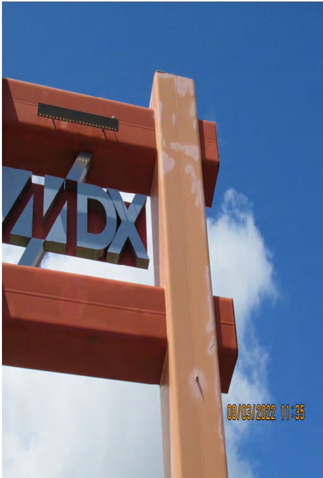
DETERIORATED PAINT ON MONOTUBE (STRUCTURE # 87A327)
