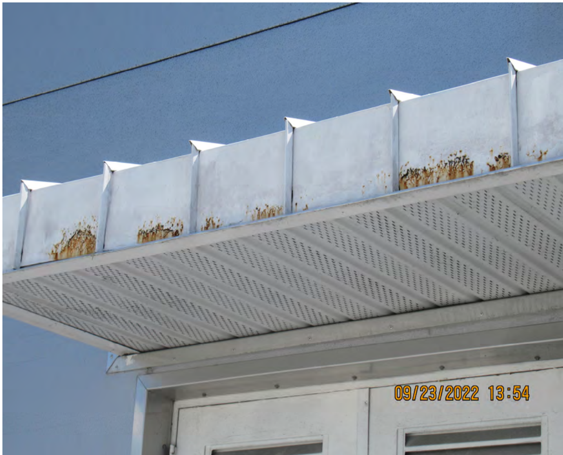
SURFACE CORROSION ON METAL AWNING
