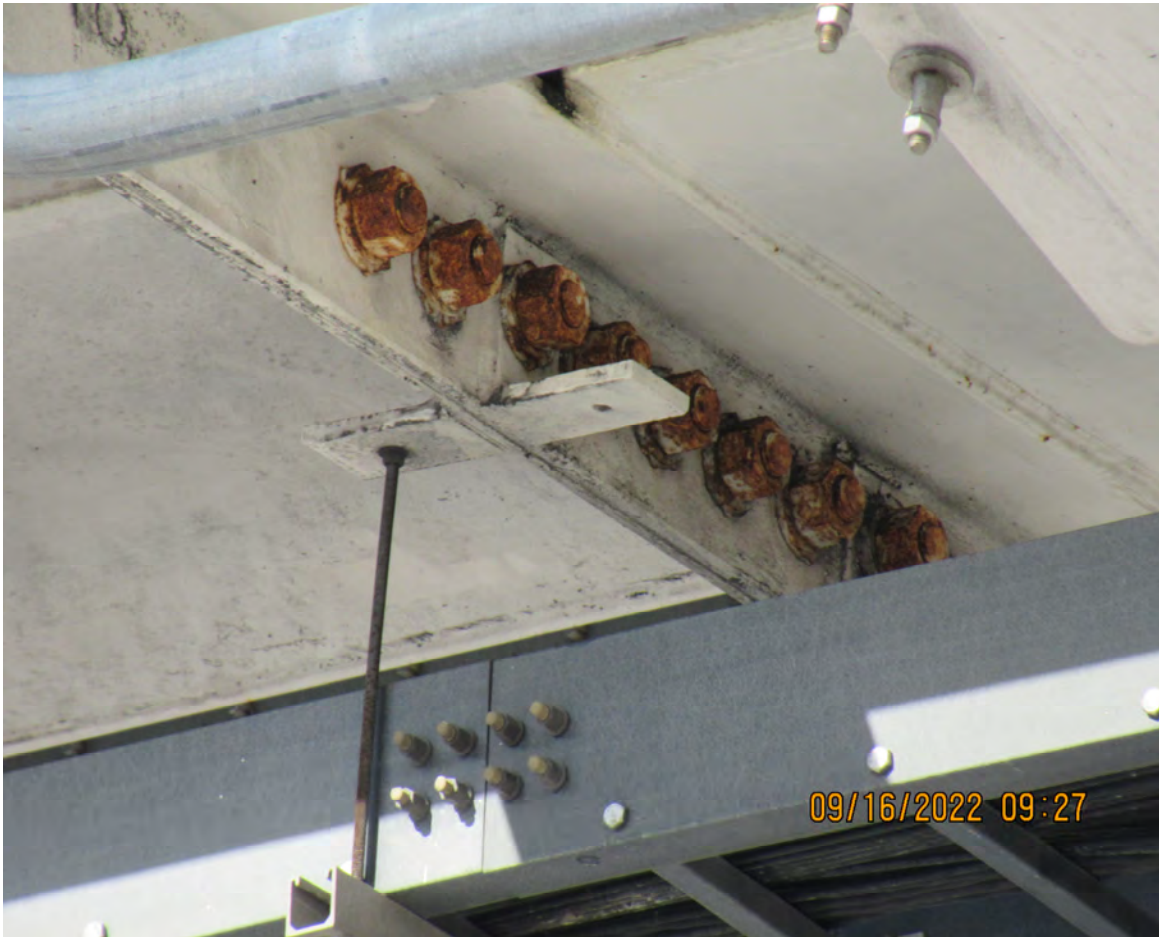
CORROSION ON ORT GANTRY BOLTS (STRUCTURE # 87A253)
