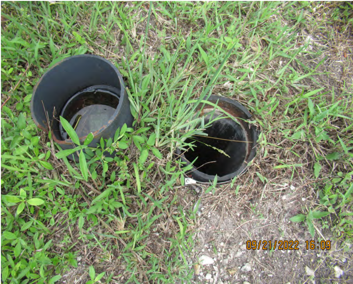
DETACHED SANITARY SEWER CLEANOUT CAP
