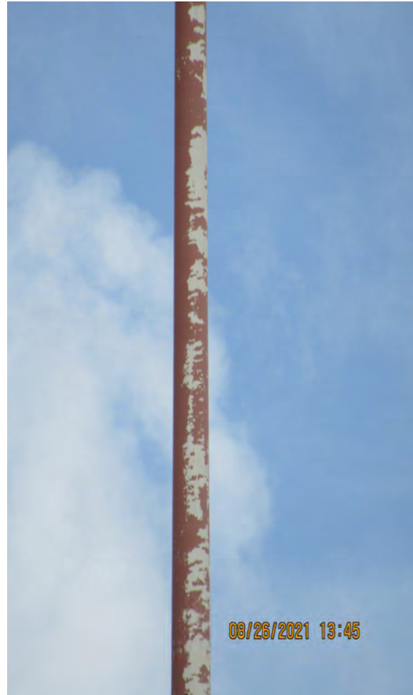
DETERIORATED PAINT ON HIGH MAST LIGHT POLE
