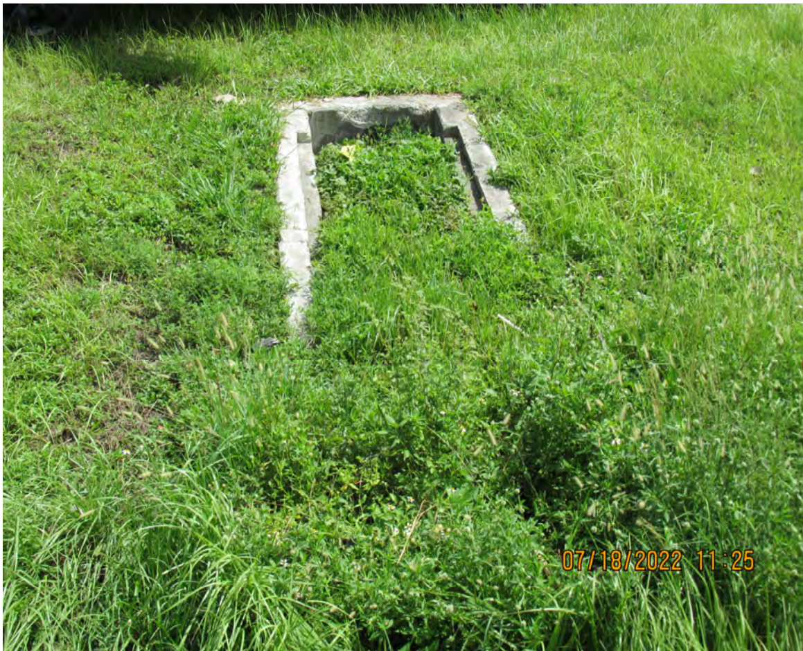
SILTED END WALL (TYPICAL TROUGHOUT THE CORRIDOR)
