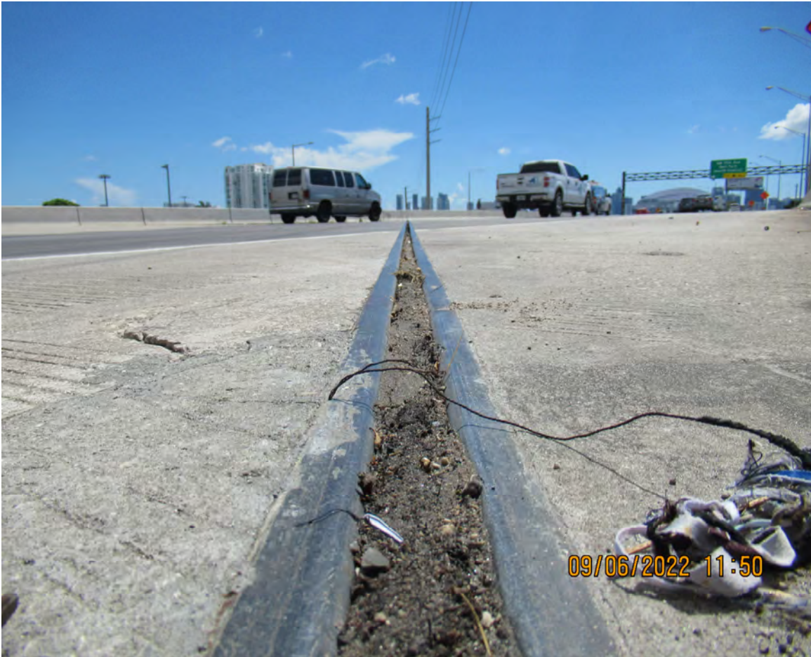
SEDIMENT AND DEBRIS ON BRIDGE EXPANSION JOINTS (BRIDGE # 870966)
