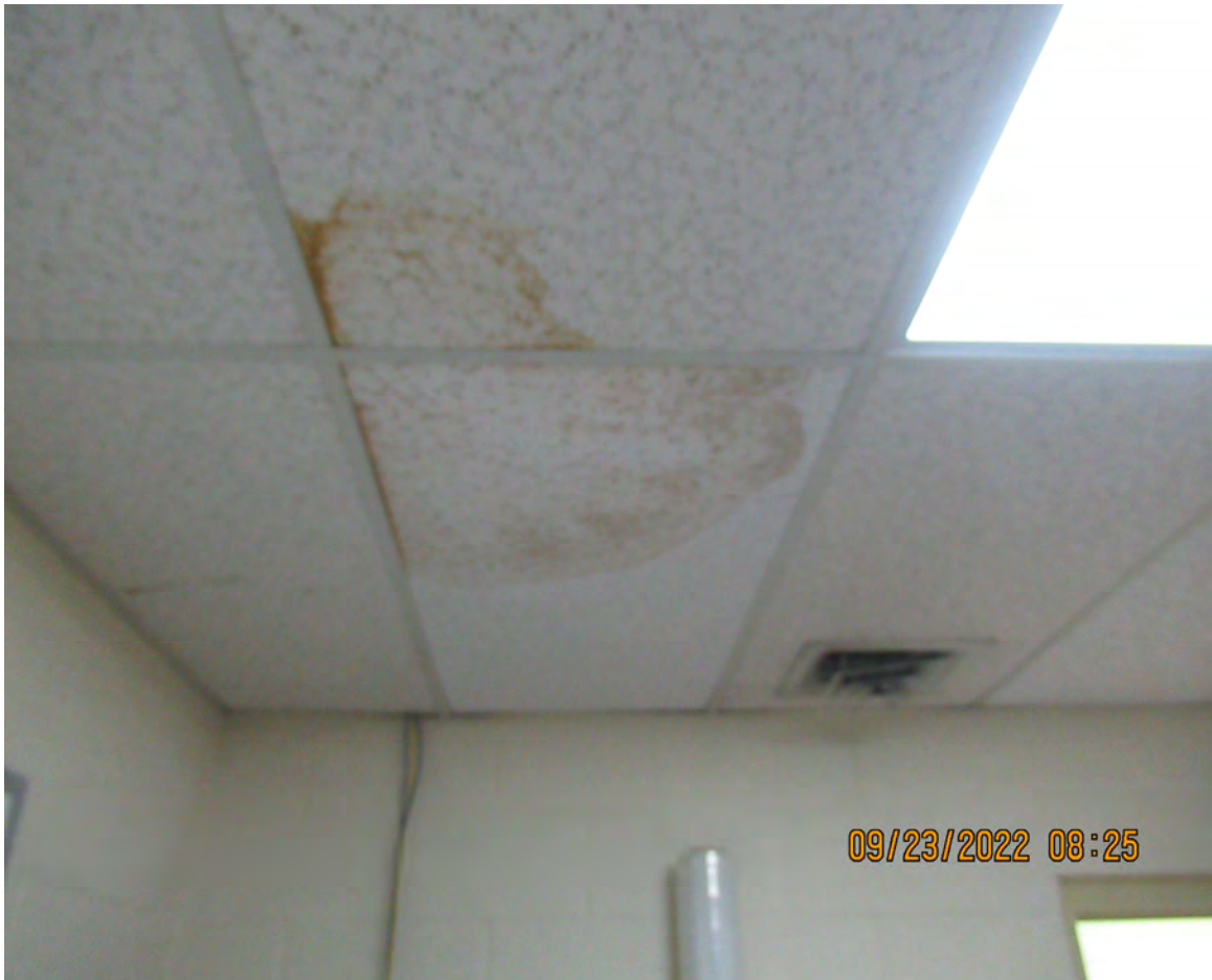
WATER STAINS ON ACCOUSTICAL TILES
