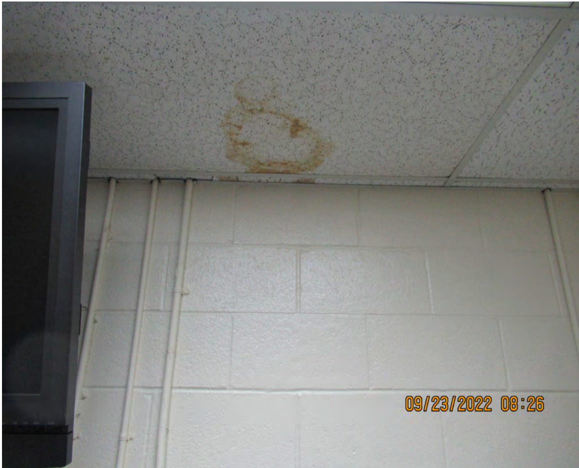
WATER STAINS ON ACCOUSTICAL TILES
