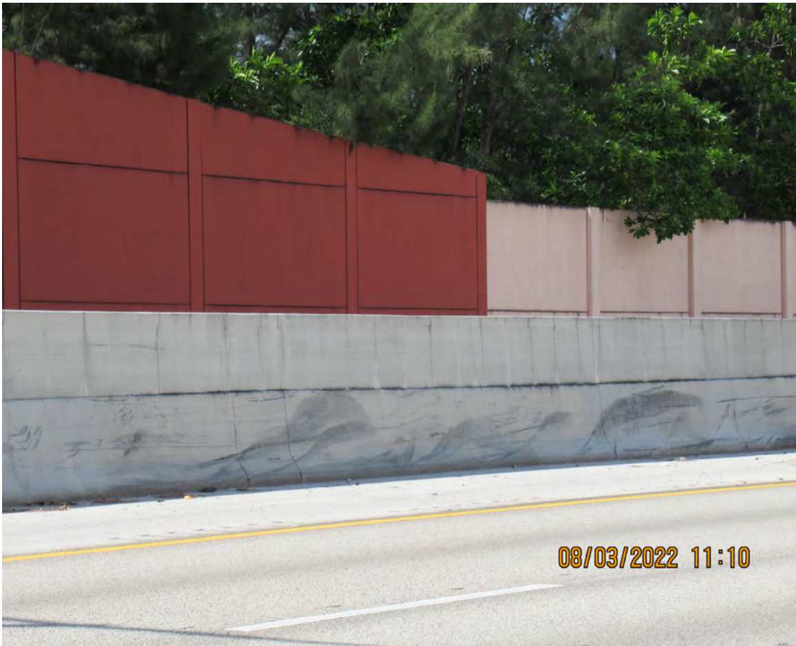
SKUFF MARKS ON BARRIER WALL (TYPICAL AT VARIOUS LOCATIONS)
